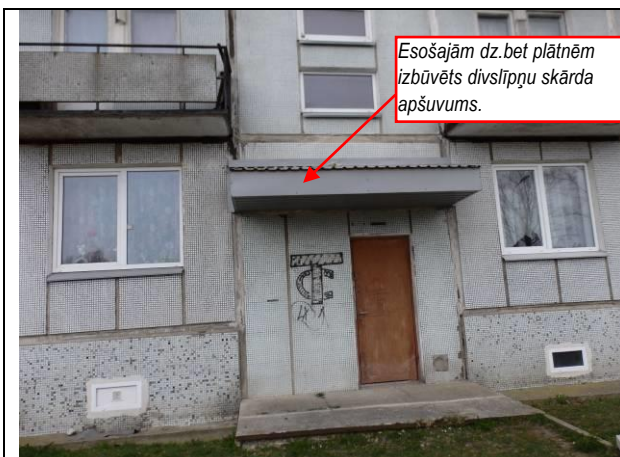
3. Austrumu fasādes fragments, atkritumu telpas durvis
